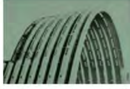
Eugene Freyssinet, Hangar in Orly 1921
